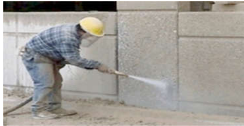
Fig: 12 Abrasive blast cleaning
