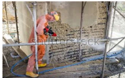
Fig: 14 High pressure water cleaning
