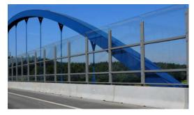
Figure No. 3 Semi-rigid barriers have two main functions:
